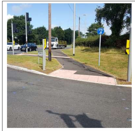
Photo 5 – Existing controlled pedestrian/cycle facility over Gravelly Way
