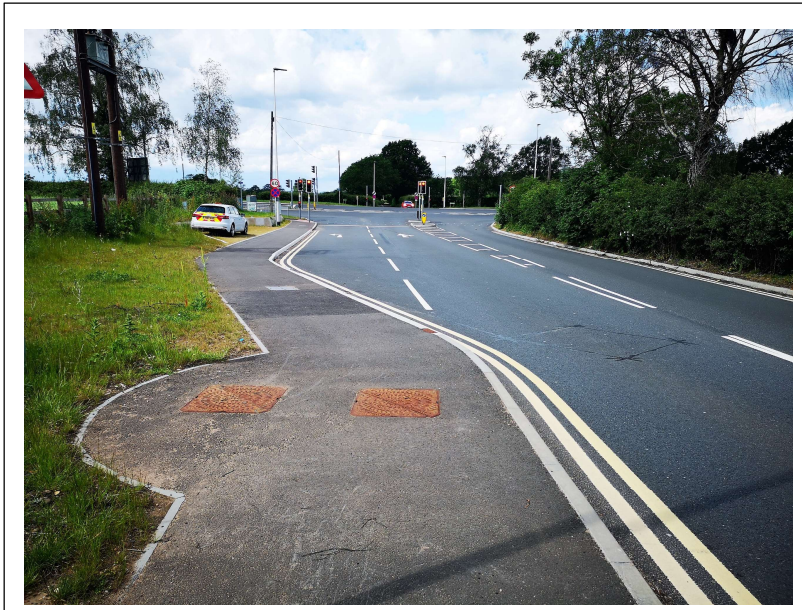
Photo 1 – View from Gravelly Way at the proposed location of the new NMU crossing.
